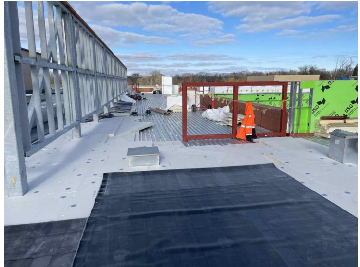
Bayside: Roofing being installed over the district office
