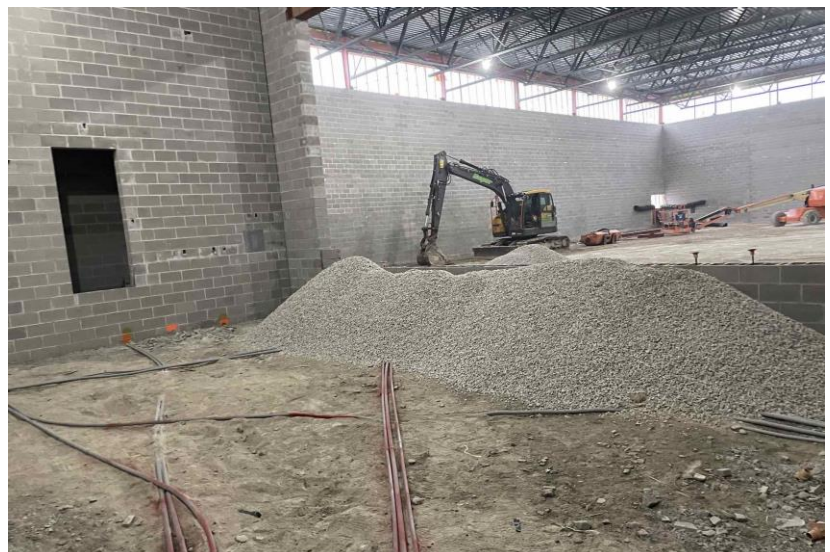
Bayside: Stage floor getting prepped for installation
