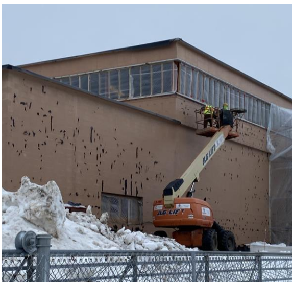
Bayside: Exterior air barrier installation
